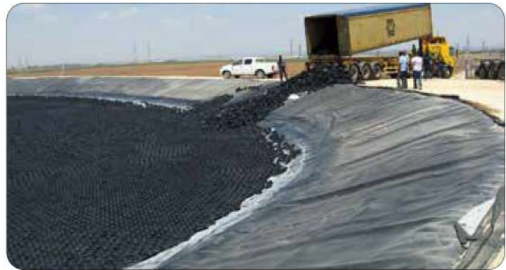
Hexa-Cover Floating Cover BULK delivery and installation:
