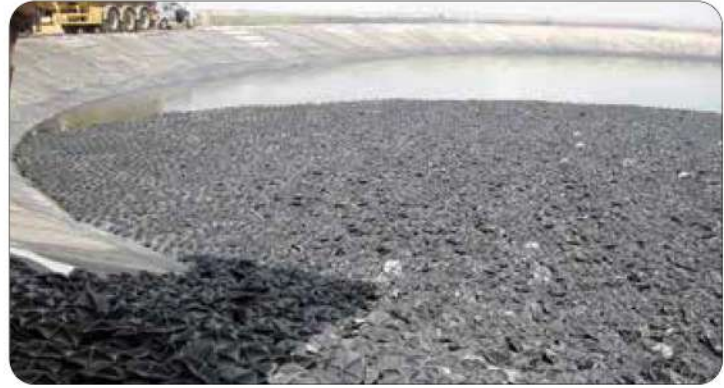
Hexa-Cover Floating Cover BULK delivery and installation:
