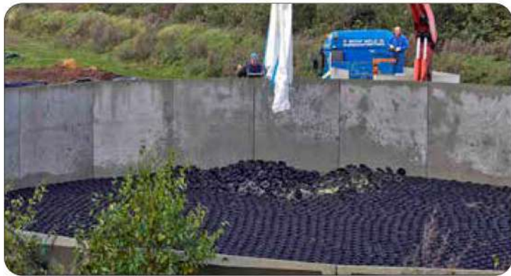
Hexa-Cover Floating Cover Big Bag delivery and installation:
