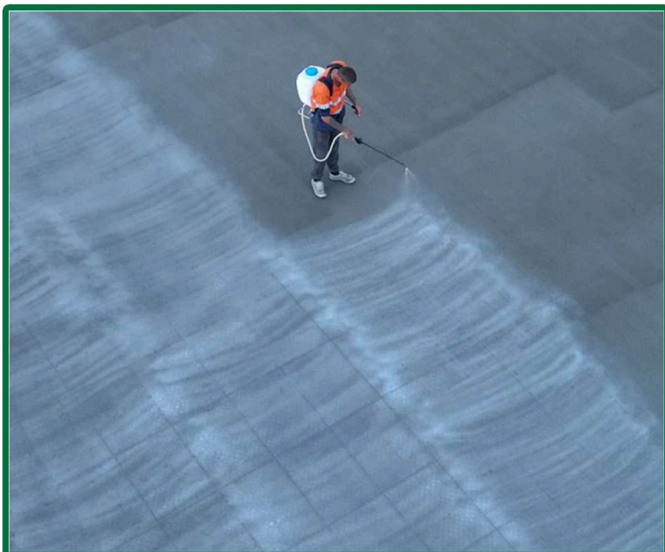
Figure 16 – A curing compound should be applied to the slab surface once installed.
