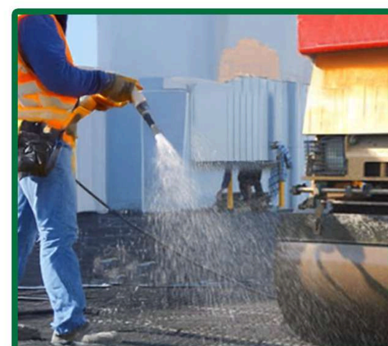
Figure 11 - Rolling in TREXLOK grid before concrete fill.
