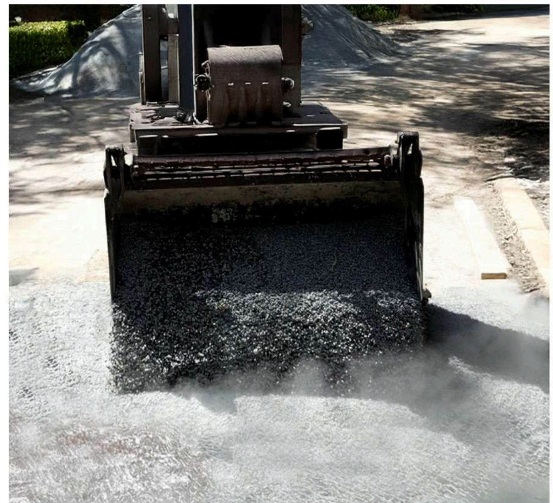
Figure 27 – Filling TREX with aggregate.
