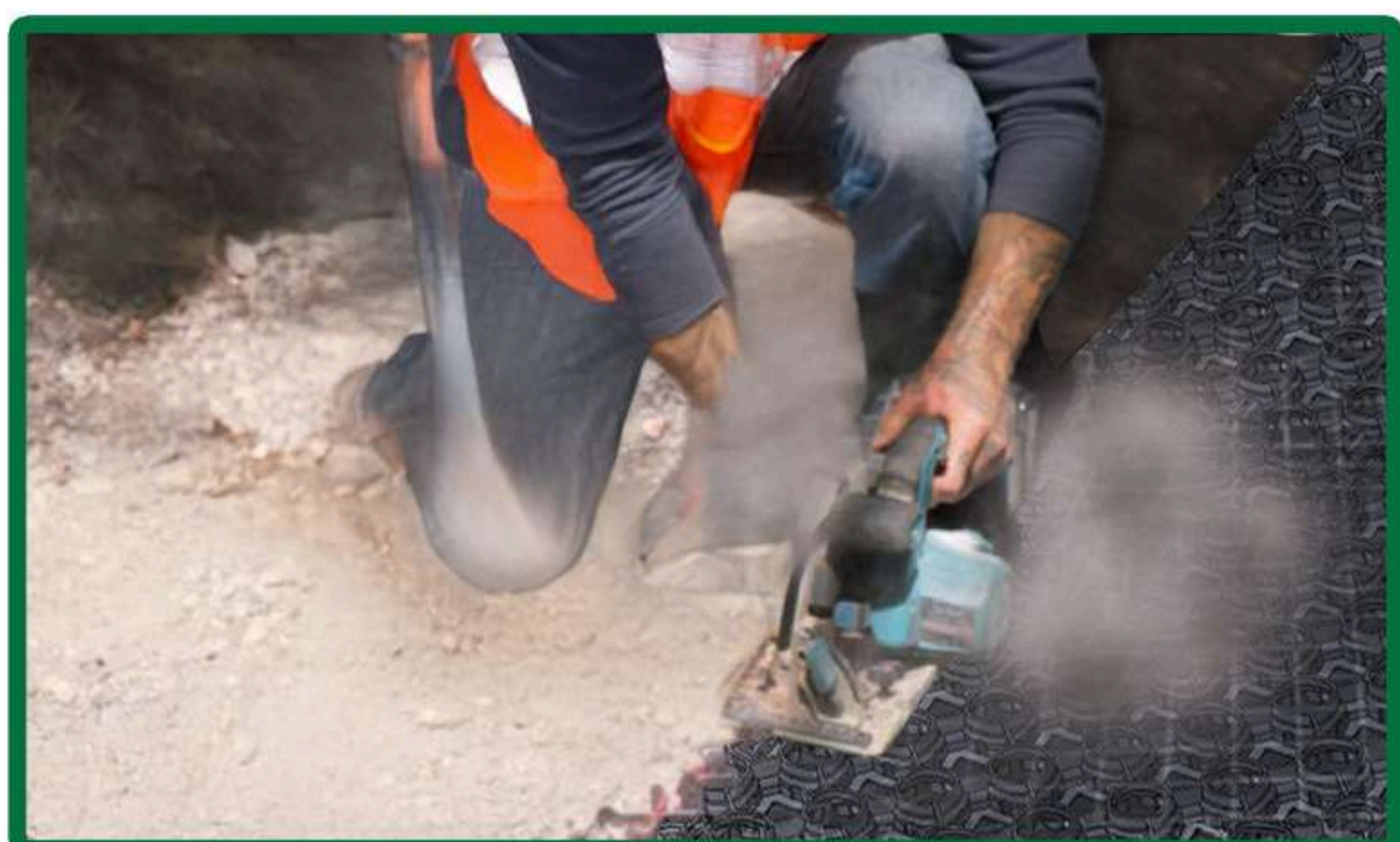
Figure 26 – TREX cut and ready for fill. Offcuts can be used on the opposite side ensuring minimum wastage.
