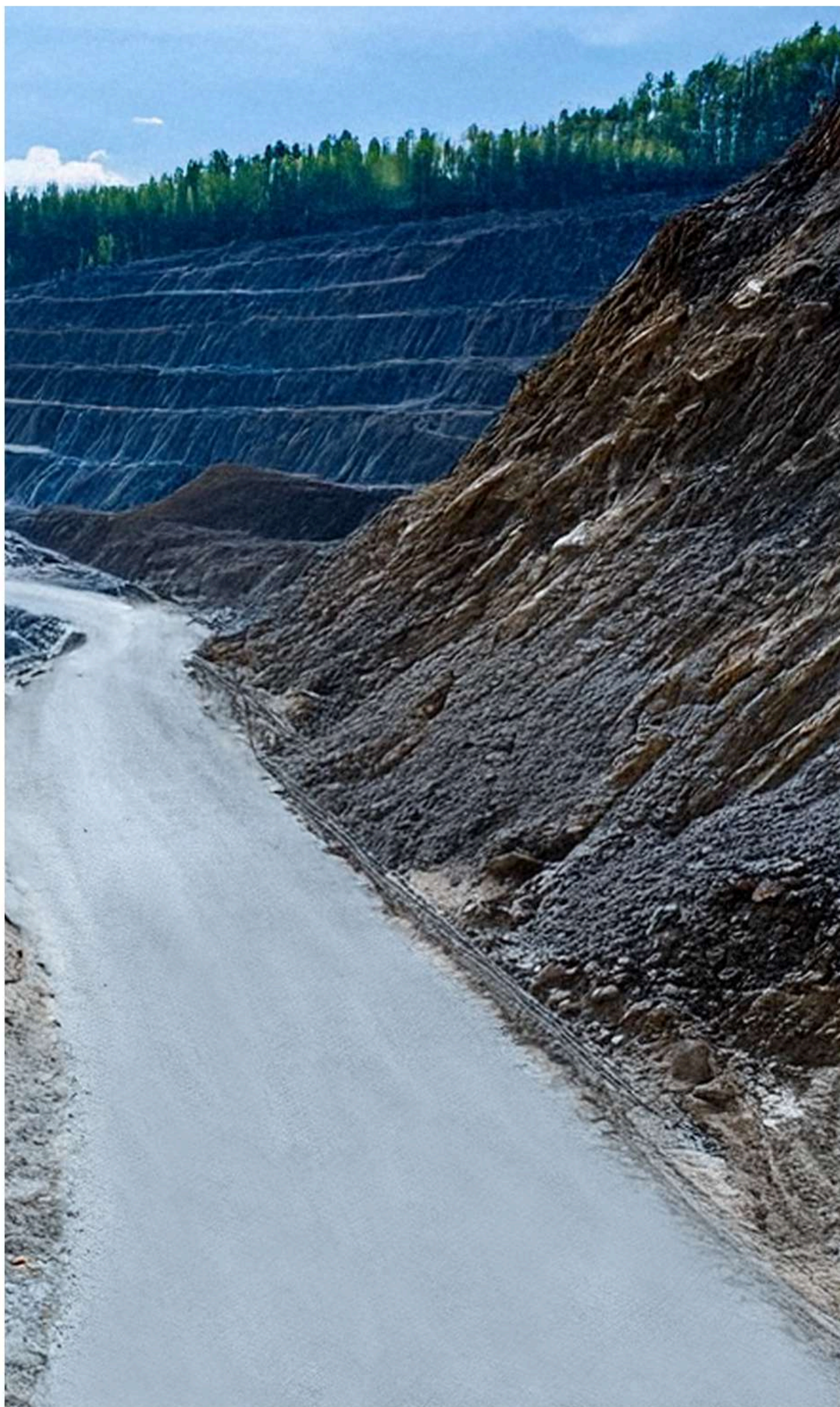
Figure 30 – Completed TREX permeable unbound pavement.
