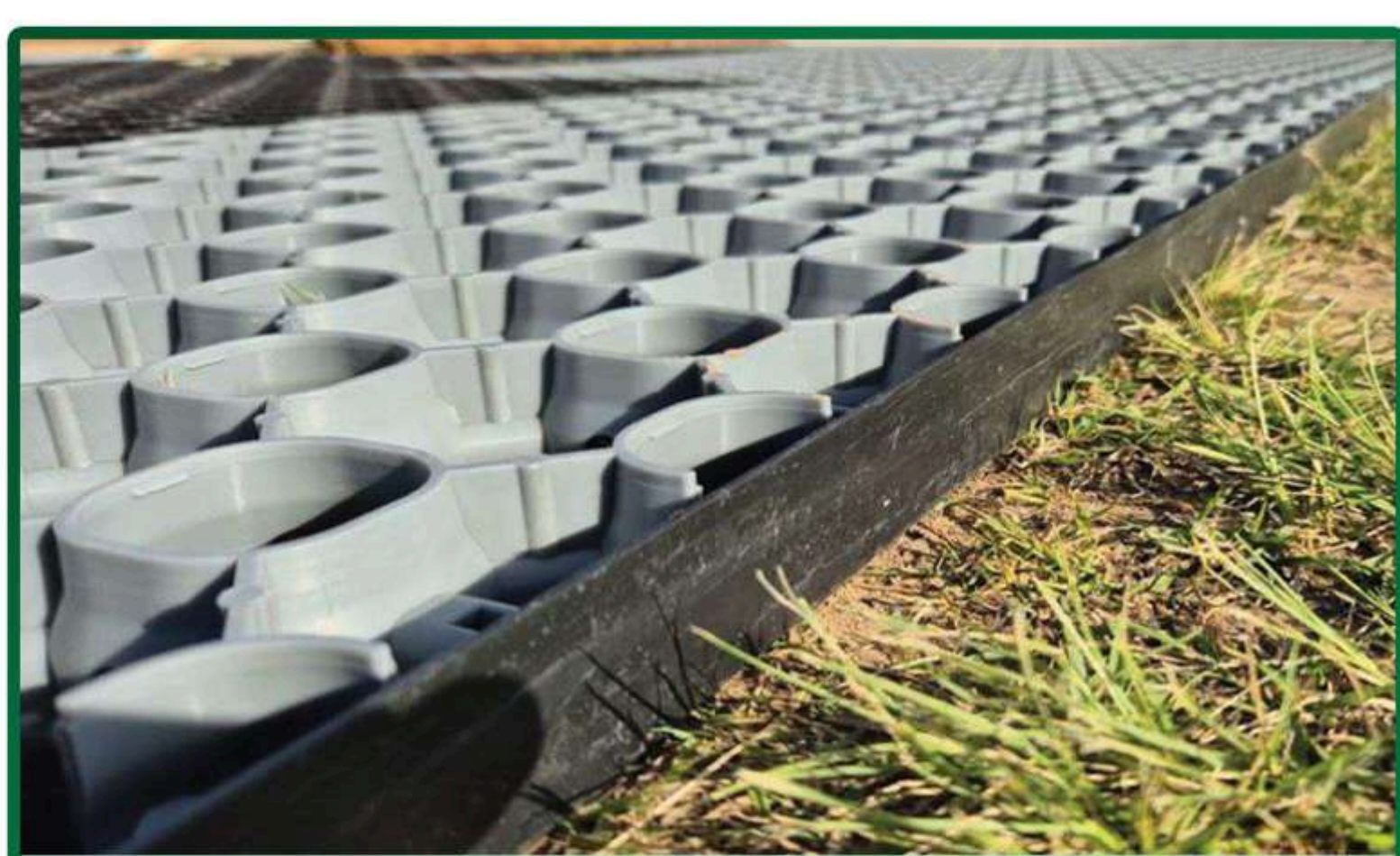
Figure 24 – Depress each connection until flat and secure.
