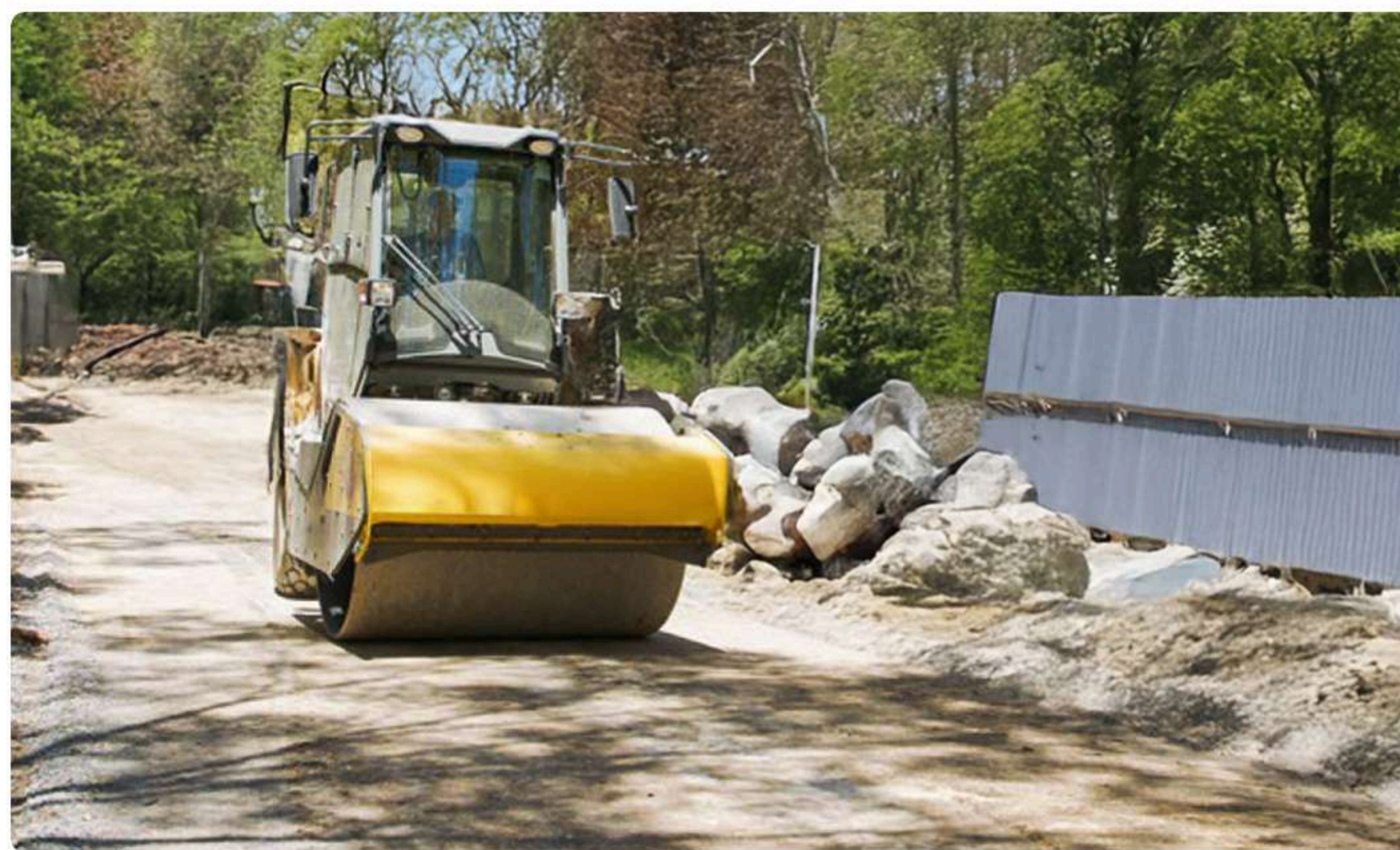
Figure 16 – Subgrade Preparation: Graded and compacted.
