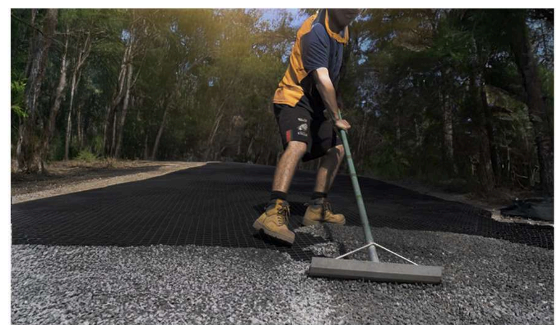
Figure 29 – Use a concrete rake to help spread evenly.
