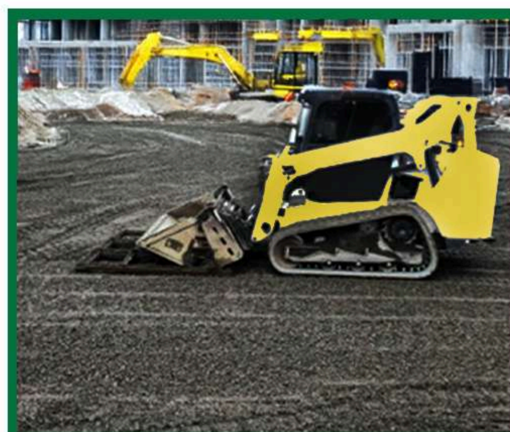
Figure 4 - Subbase Preparation: Spreading and leveling road base prior to compaction. Compacted and watered, ready for TREXLOK installation
